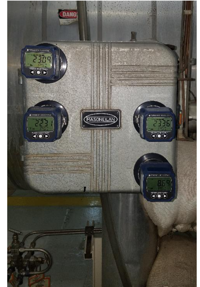
“Digitized” Pneumatic Controller
